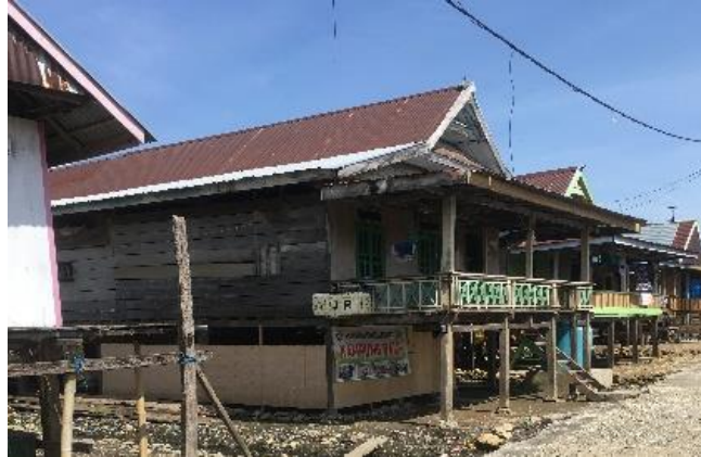
Picture. 18. Condition Buildings in Residential Pattern Areas group
