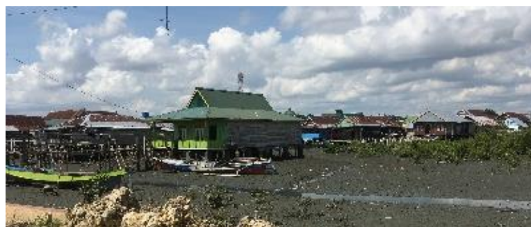
Figure 5. 2, Condition Buildings in Settlement Patterns Spread Source: Author's Analysis, 2021
